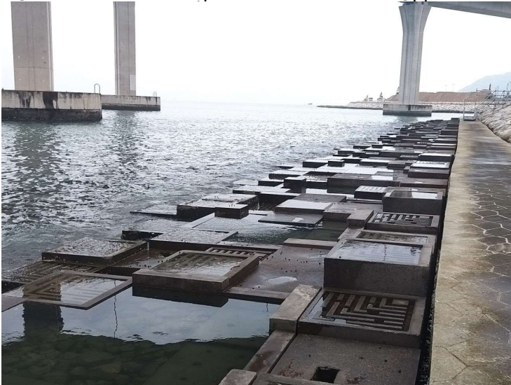
General View of Rocky Eco-shoreline
